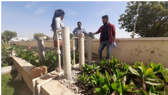
Constructed Wetland for treatment of domestic wastewater from residential area (NIH Colony Roorkee)
