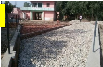
Constructed wetland under progress
